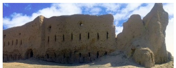
Figure 2. A general view of "Gavur Kala"
